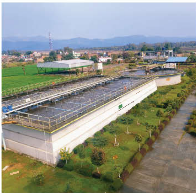
4 MLD CETP for Industrial Area, Sitarganj, Uttrakhand
