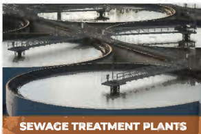
SEWAGE TREATMENT PLANTS
