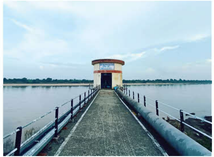
Rural Water Supply Project, Sehore, Madhya Pradesh
