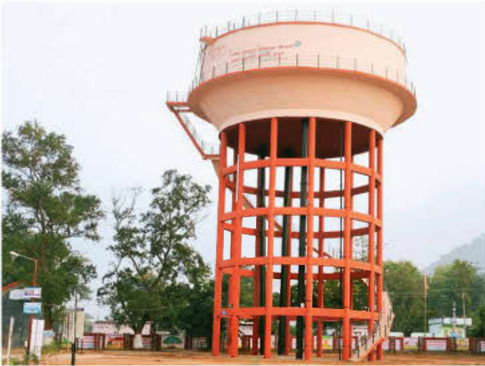
Elevated Water Reservoir
