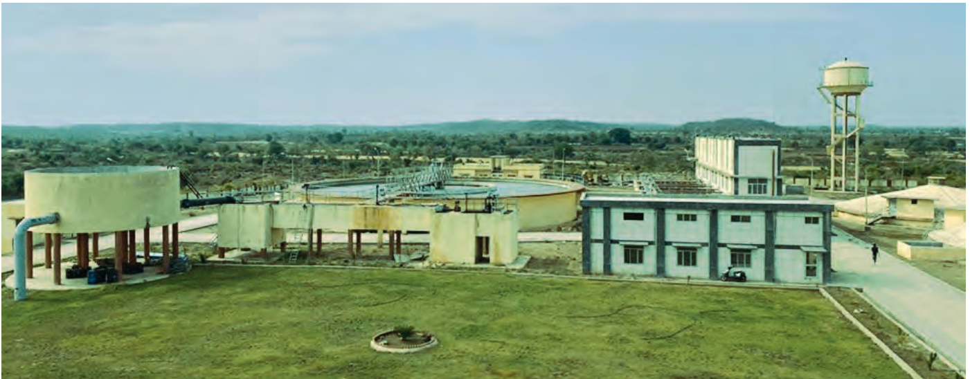
Gagreen Water Supply Scheme, Rajasthan
