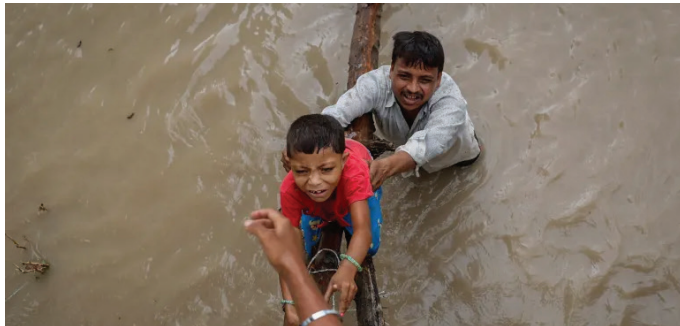
A man helps his son to climb onto a flyover under construction after being displaced by the rising water level of the Yamuna River in New Delhi [Adnan Abidi/Reuters]
