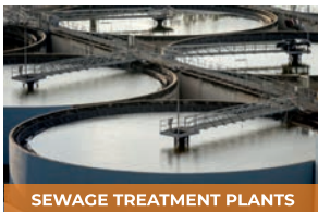
SEWAGE TREATMENT PLANTS
