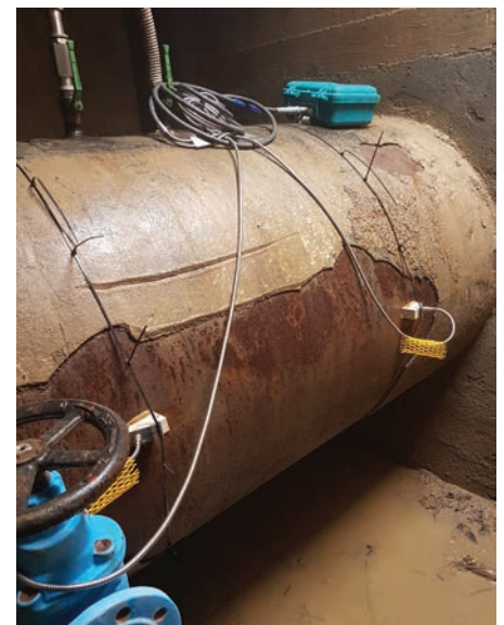
Courtesy: The digital twin provides a single source of truth for the owner, improving decision-making and driving smart water management over the next 30 years. Image courtesy of Hidroing d.o.o.
