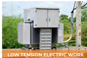
LOW TENSION ELECTRIC WORK
