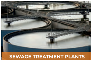
SEWAGE TREATMENT PLANTS
