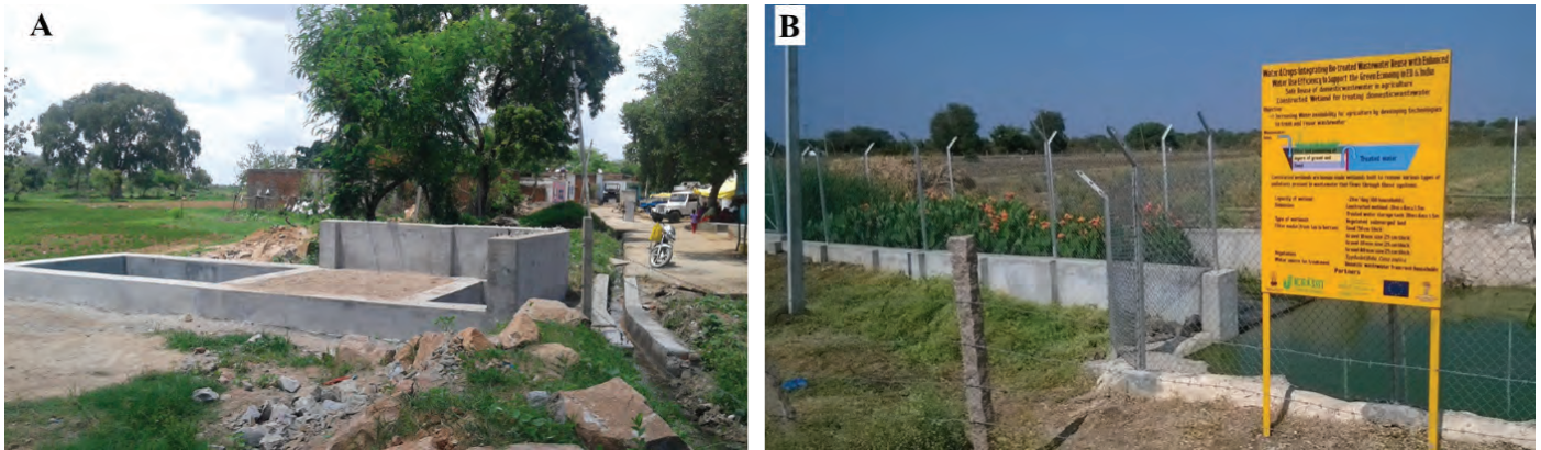
Figure 2: Constructed wetland implemented in Dhikoli (A) and Kothapally (B) (Source:15)
