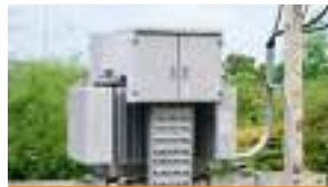
LOW TENSION ELECTRIC WORK
