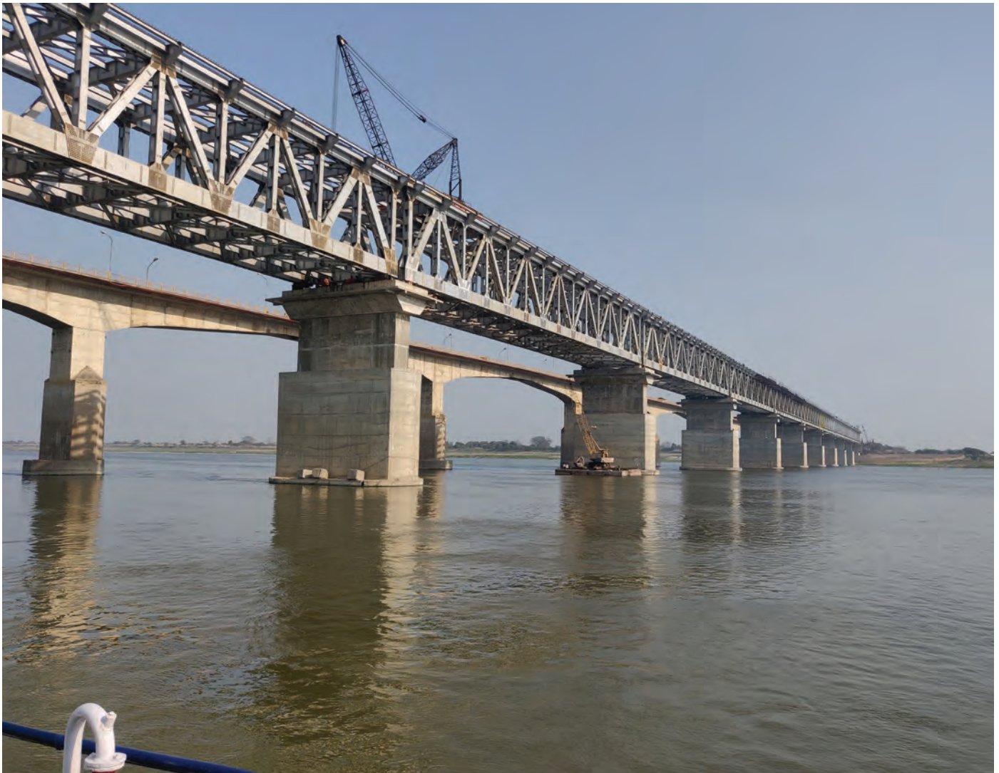
Figure 1 River Over Bridge (Ghazipur, UP © Floodkon Consultants LLP)
