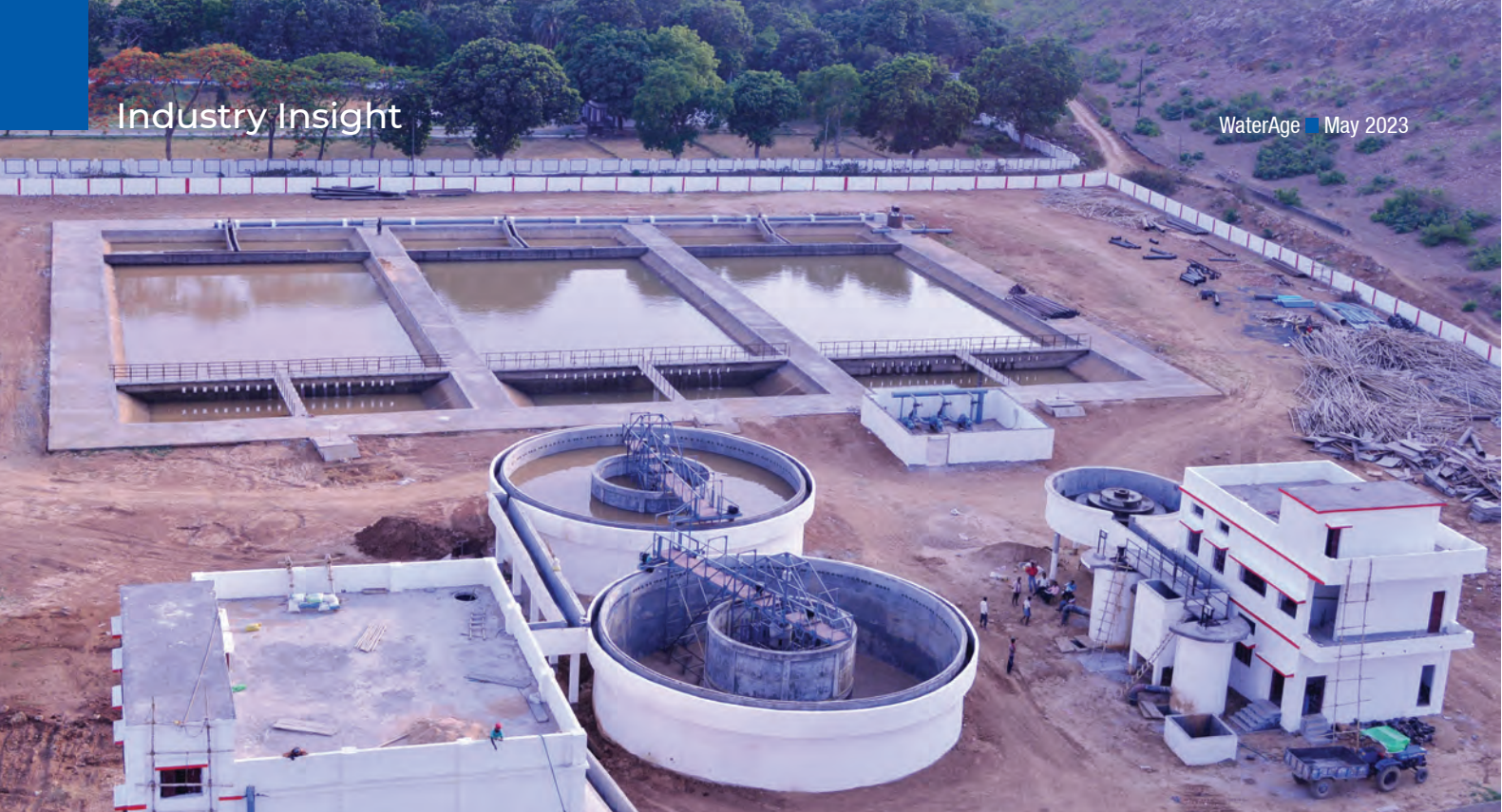
6.5MLD Water Treatment Plant, Munger, Bihar
