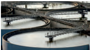
SEWAGE TREATMENT PLANTS
