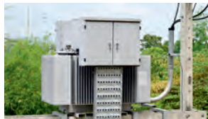
LOW TENSION ELECTRIC WORK
