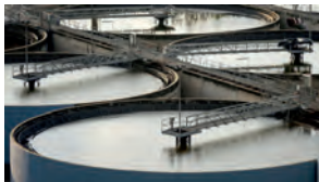
SEWAGE TREATMENT PLANTS
