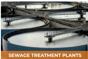
SEWAGE TREATMENT PLANTS
