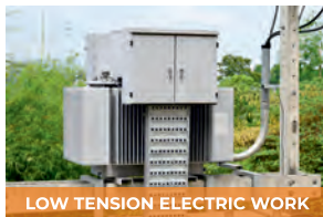
LOW TENSION ELECTRIC WORK
