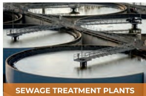
SEWAGE TREATMENT PLANTS
