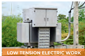
LOW TENSION ELECTRIC WORK
